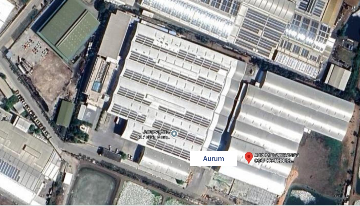
Factory size: 54,400 sqm with 0.66MGW solar energy
